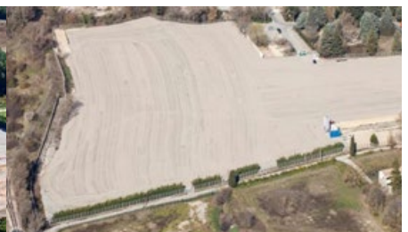
After the works (2017)
