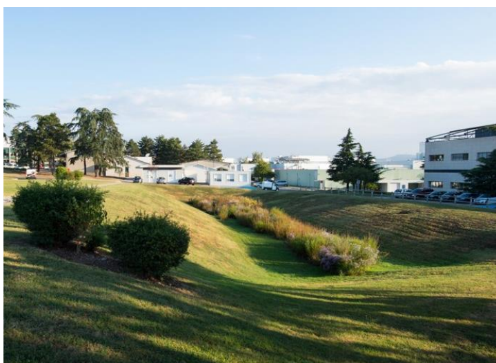
Stormwater basin Marcy-l'Etoile, France. 2020
