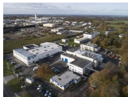
Overview of Sanofi site in Ploërmel
